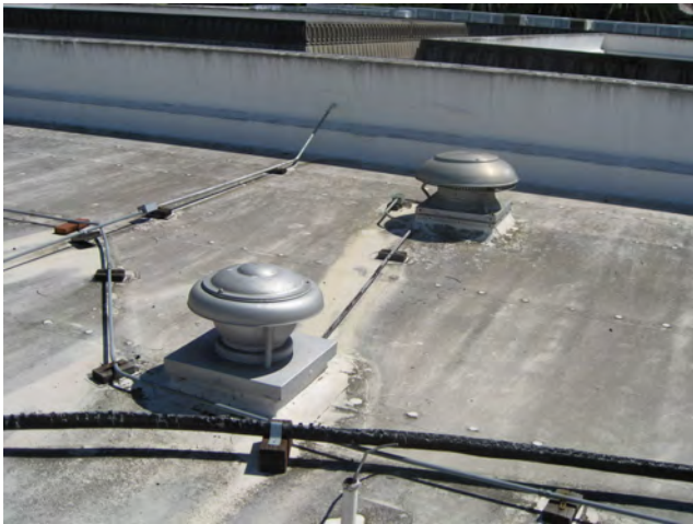
Typical older rooftop exhaust fans
