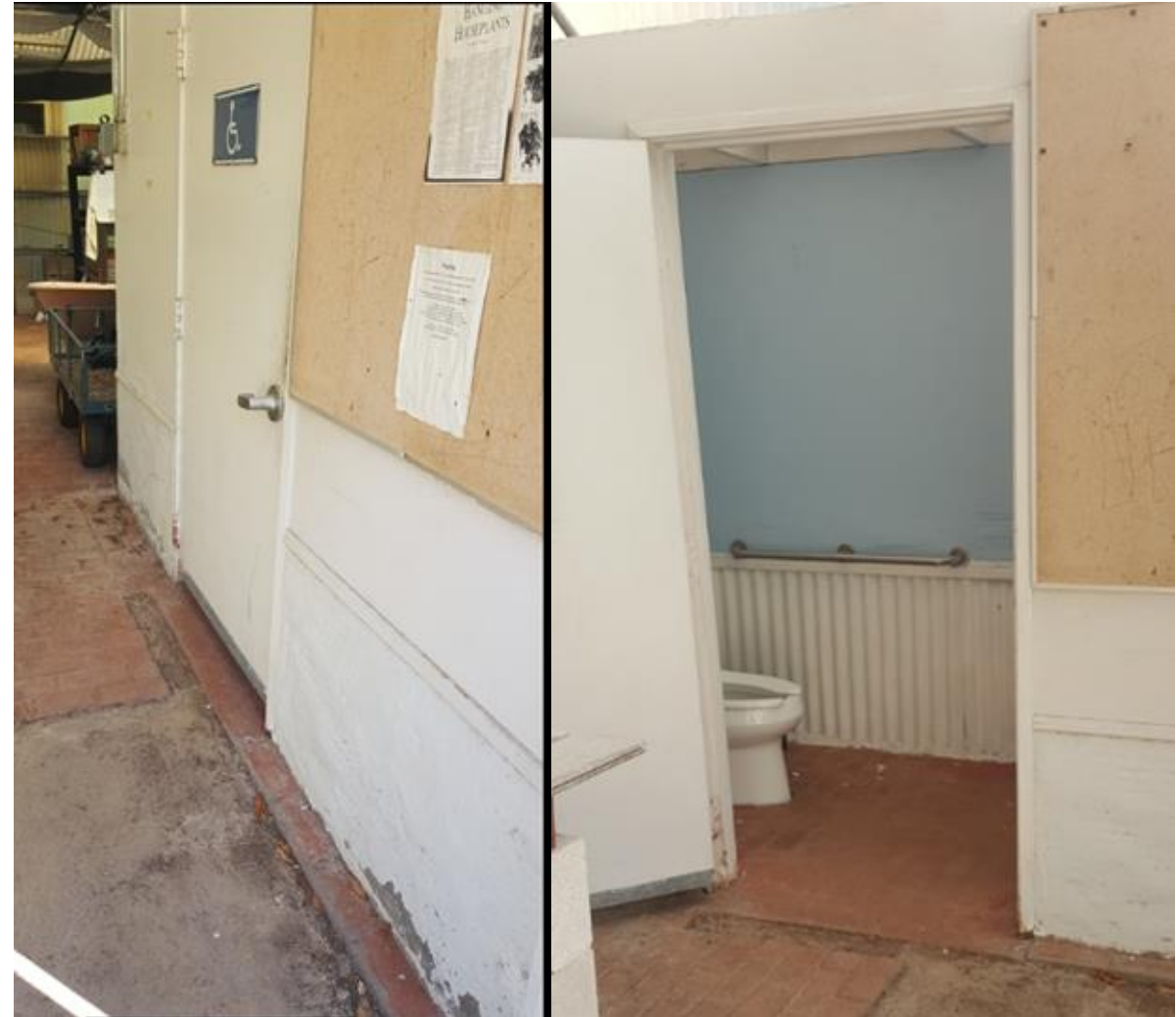
Current condition of restroom
