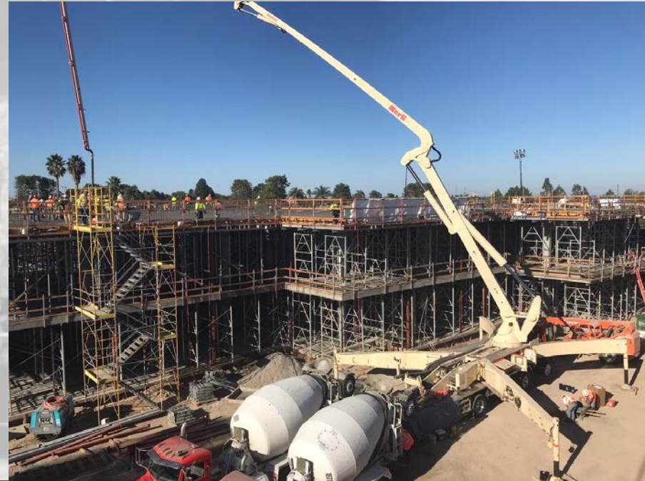
Concrete placement
